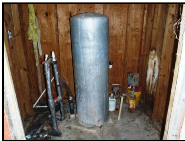
Photo of the well pump station
